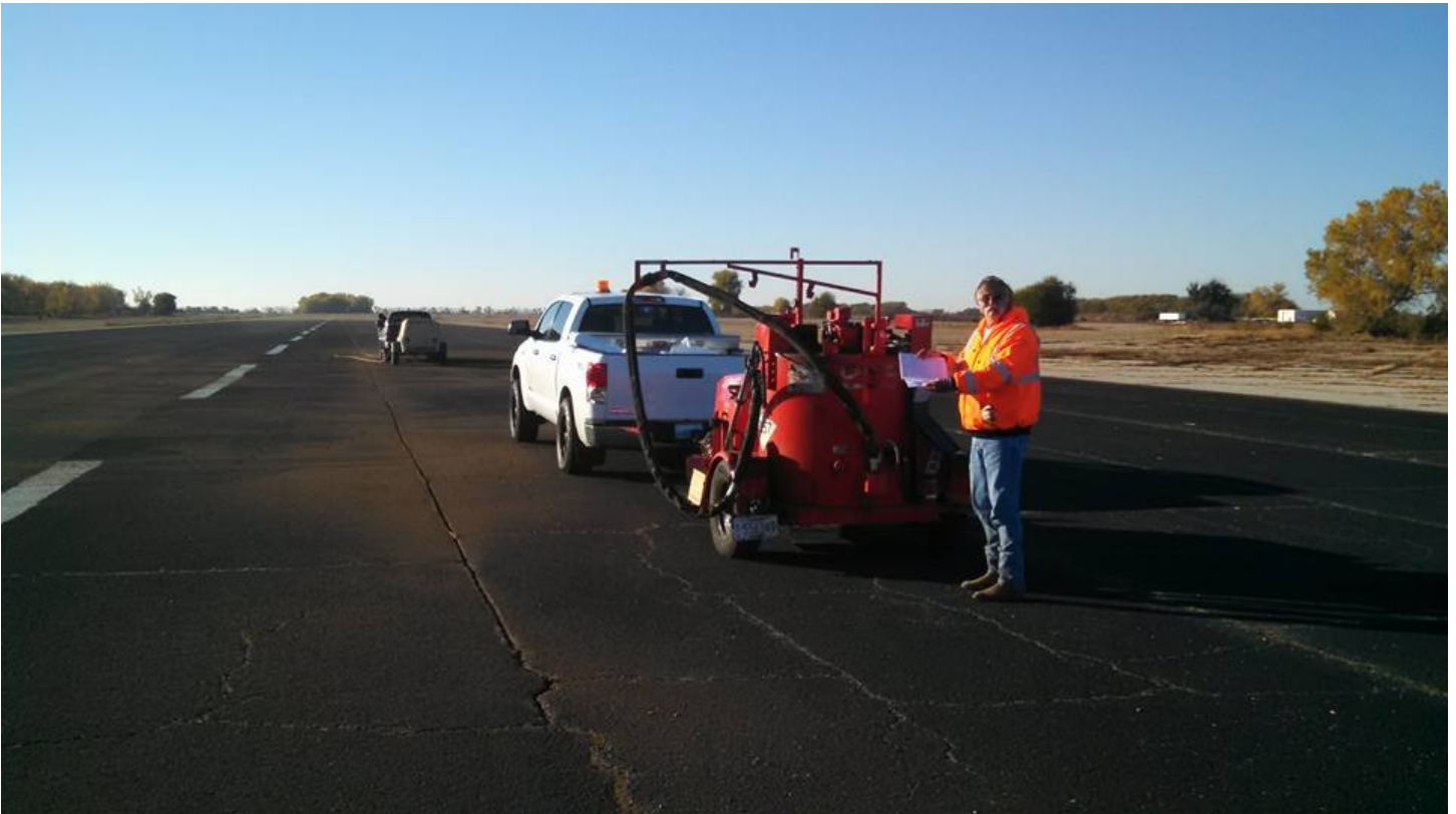
Mike Davis sealing cracks on the runway
